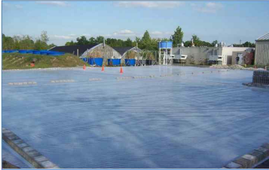
Figure 5. Parking lot covered in plastic sheeting for rainwater collection.
